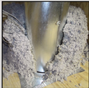
VARIED DEPTH OF CELLULOSE INSULATION
