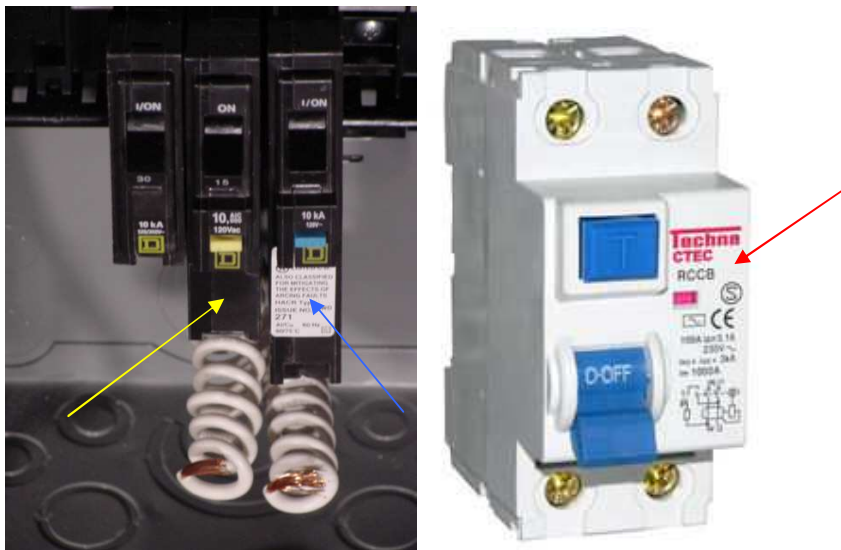
Fig. 6 and 7, GFCI (yellow arrow), AFCI (blue arrow), and RCD (red arrow), Schneider Electric SA.
